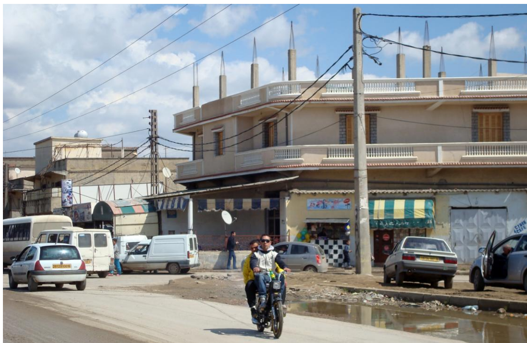
Figure 3 – Iron rods waiting for future extensions, bare walls, and unfinished buildings give an impression of building work in progress. Source: Troin, 2009.
