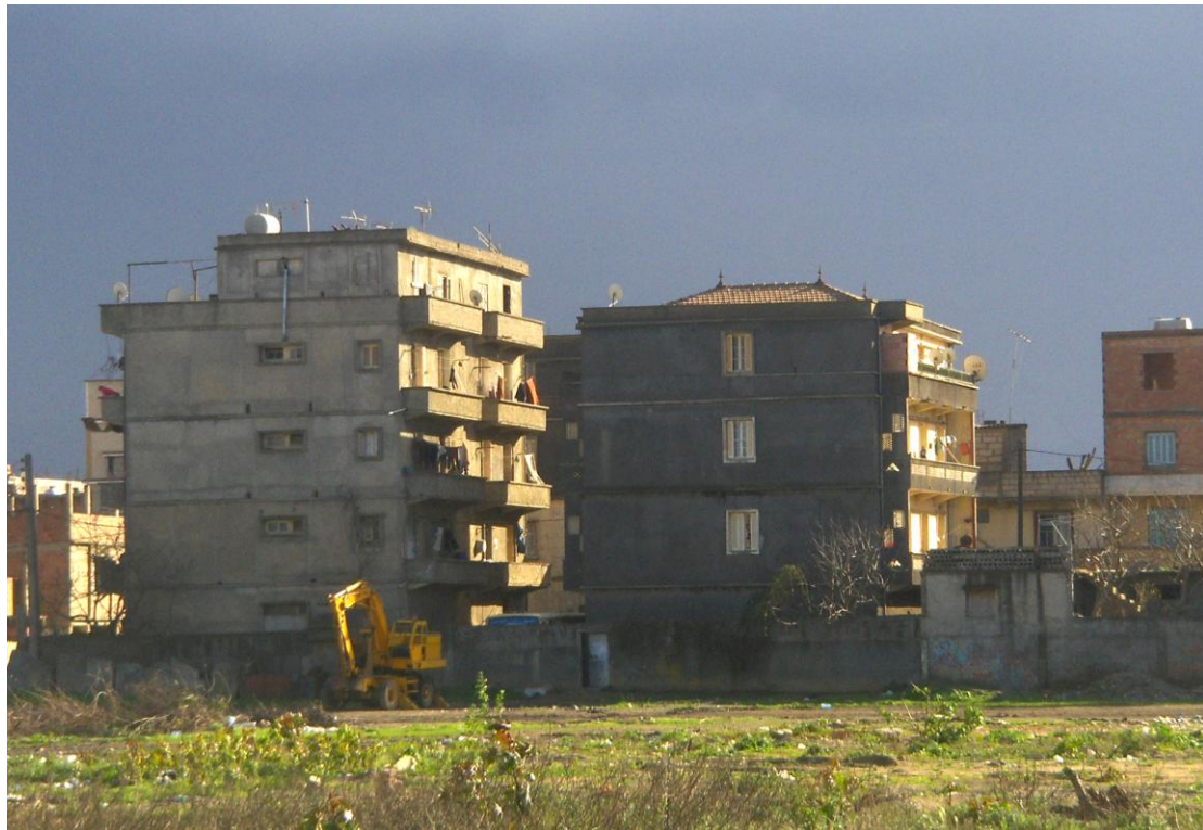
Fig. 9 - Poclain digger lent to the inhabitants by the municipal council.
