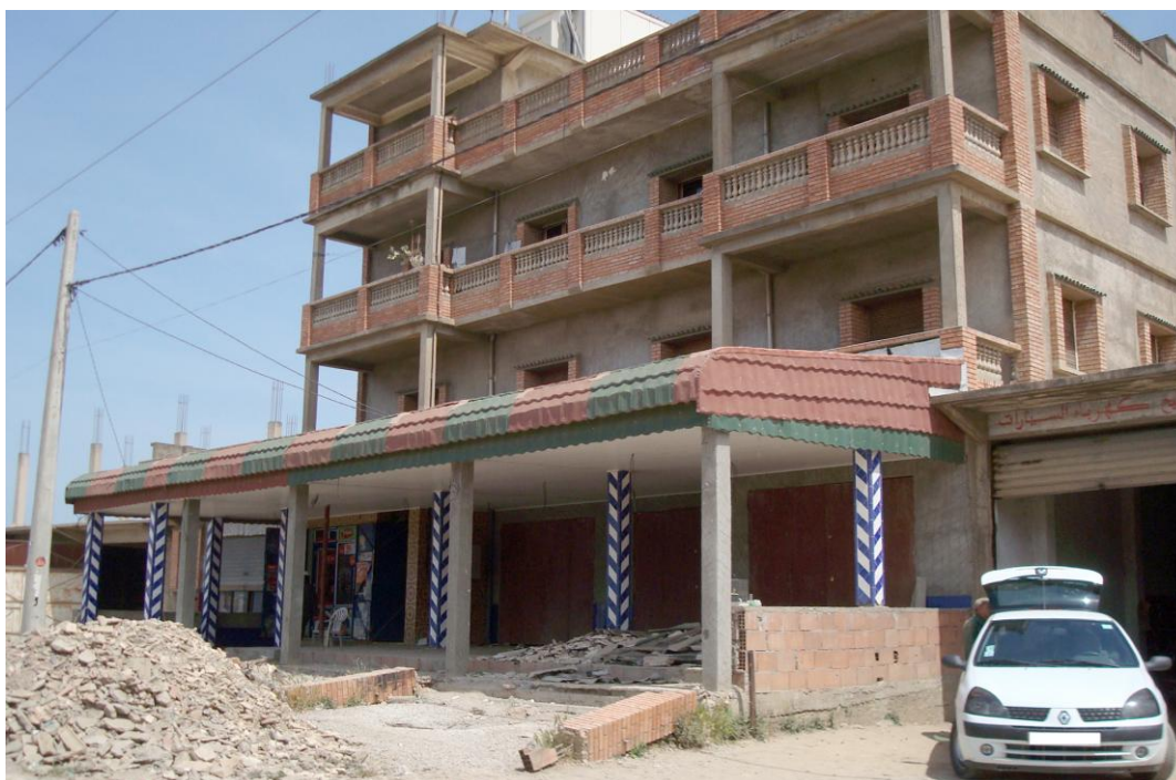
Fig. 2 – The family building: apartments on several floors are occupied by family members.
