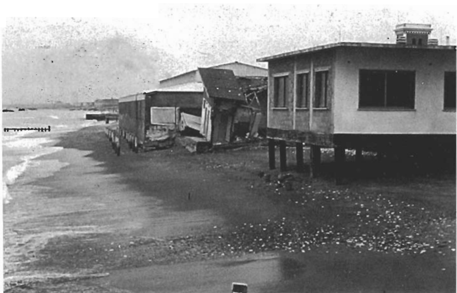
FIG. 7 – SHORELINE EROSION ON AN URBANISED COAST (LATIUM).
