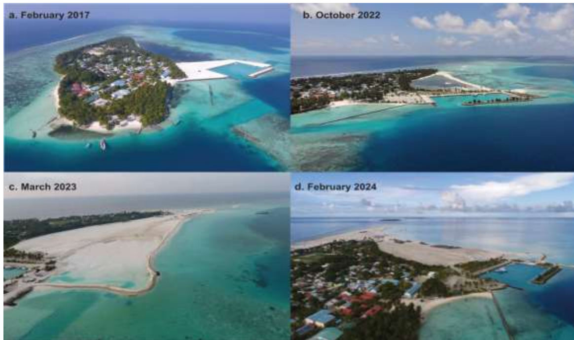
Figure 3. Overview of Magoodhoo from drone images highlighting the various stages of land reclamation around the island. (a) provides an overview of the entire island in 2017, clearly showing the bare land resulting from the initial reclamation for building the harbour (2016/2017). Images (b), (c), and (d) highlight the various stages of the reclamation process from October 2022 to February 2024. Source: elaborated by Fallati.
