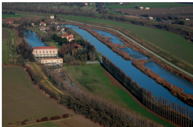
Figure 5. Bonifica Renana water-pumping plant and artificial channels. Headquarters of the Land Reclamation Museum. Source: Sergio Stignani.
